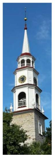
It is time to repair and restore the historic and iconic clock tower, complete with the belfry, lantern, and spire of Trinity Chapel. Dry rot and decay, both natural byproducts of age, along with water damage and weathering over the years, require restoration. The estimate for repair is \$1,000,000.
